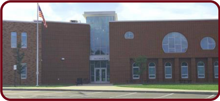
McCormick Middle School 627 North Main St., Wellington, Ohio 44090
